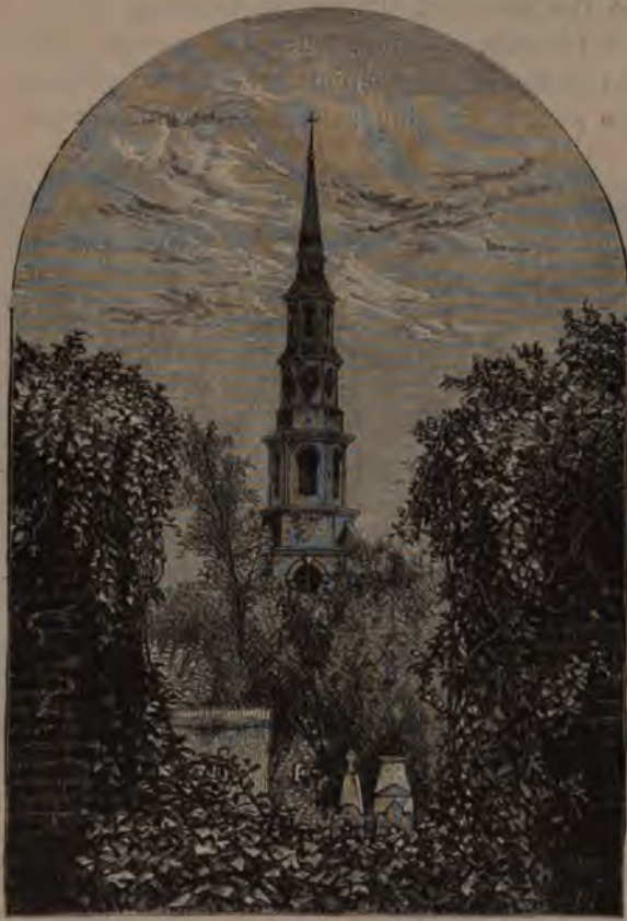
The Spire of St. Philip's Church—Charleston.
